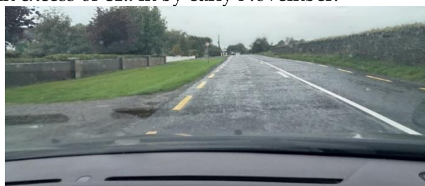
New pavement on N77 near Clintstown
