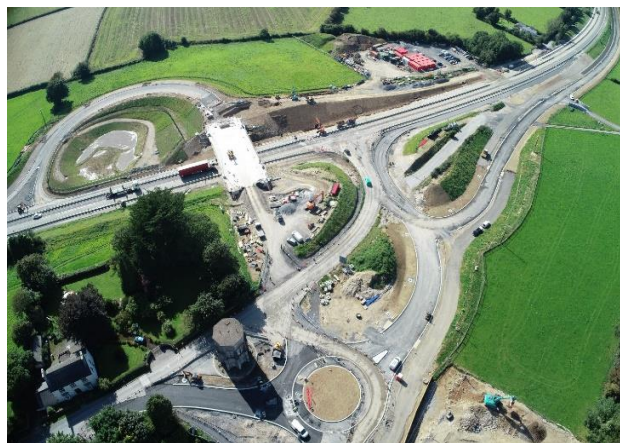
Overhead drone footage of the compacted grade separated junction under construction.
