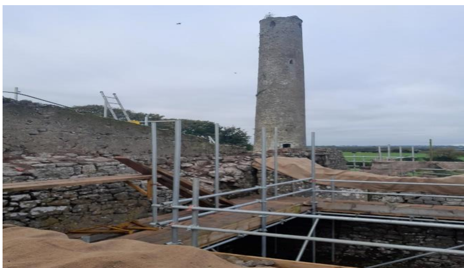
Ongoing site works at Grangefertagh
