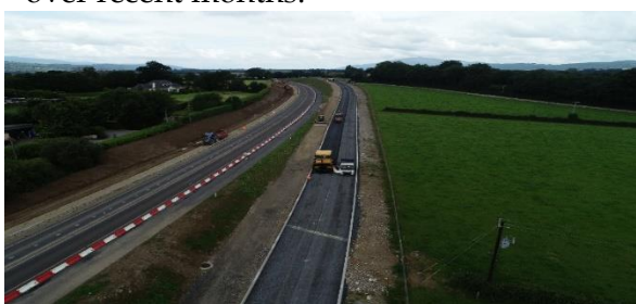
Pavement Works on-going on the Mainline and Link Road.
