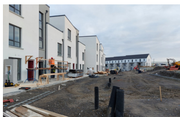
Works ongoing on Pennefeather Green Hebron Road
