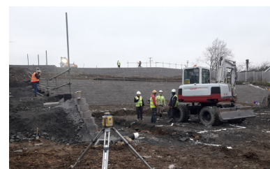
Site Development Works at Ladywell Thomastown
