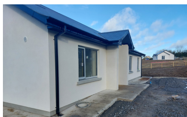
2 houses at Shanganny Jenkinstown almost complete.
