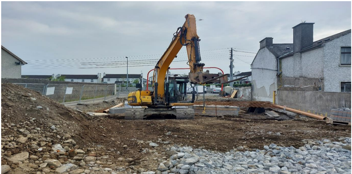
Work Progressing on Golf Links Road – 6 units – infill scheme
