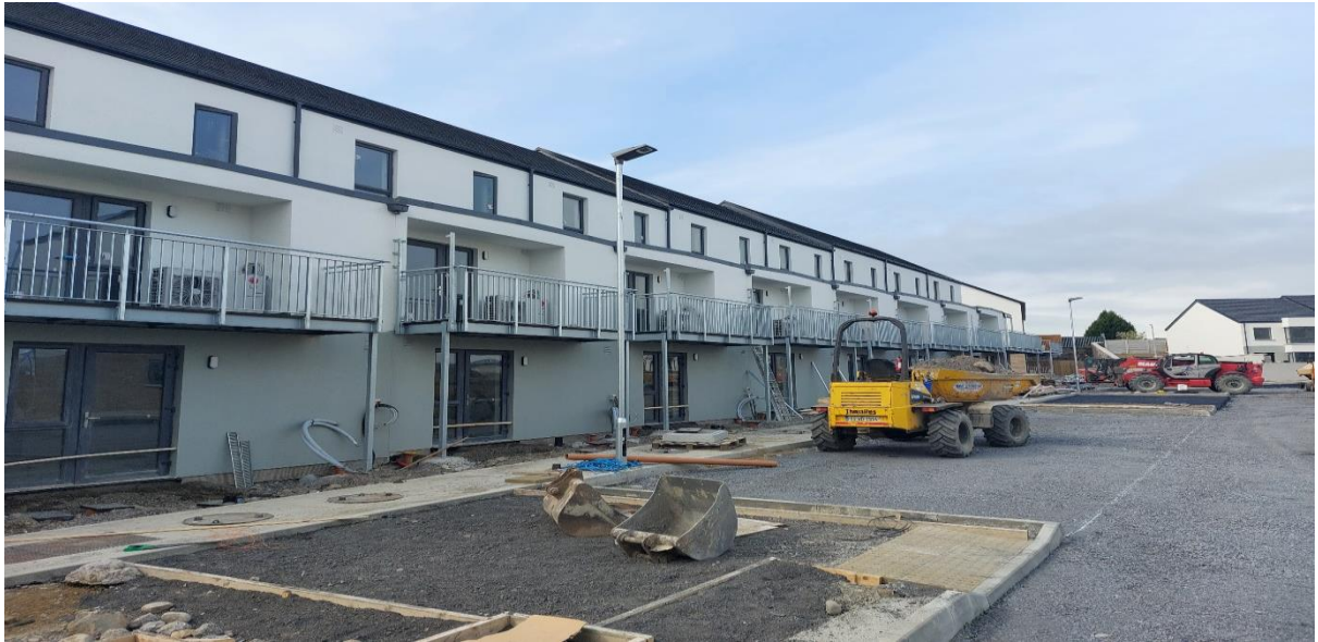
Works on Pennefeather Green nearing completion
