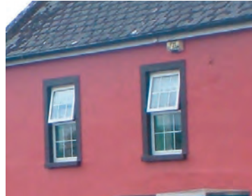
uPVC windows following traditional positioning and shape
