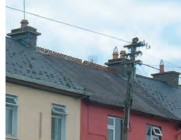
Traditional roof coverings and chimney stacks
