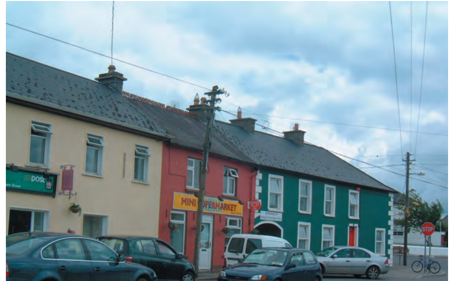
This row of shops retains traditional roofs, chimneys and painted finish
