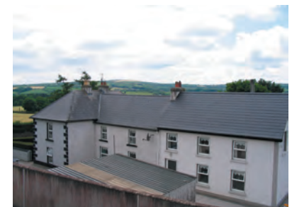
Building with traditional features
