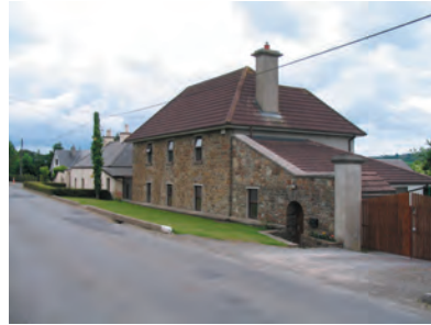
Half-hipped roof on detached house
