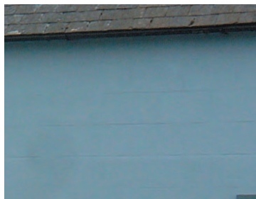
Simple painted brick and render finishes
