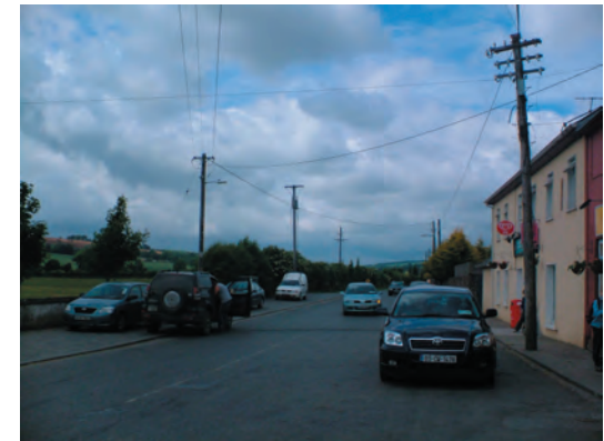
Re-routing of overhead cables could improve the appearance of the village
