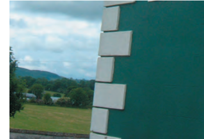
Decorative quoins on building corners
