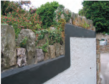
Frontage walls and boundaries
