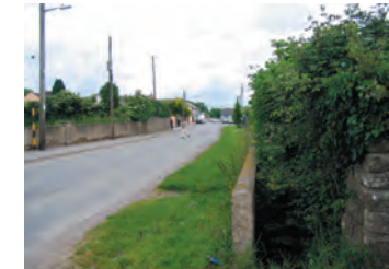
6 View from north approach road.
