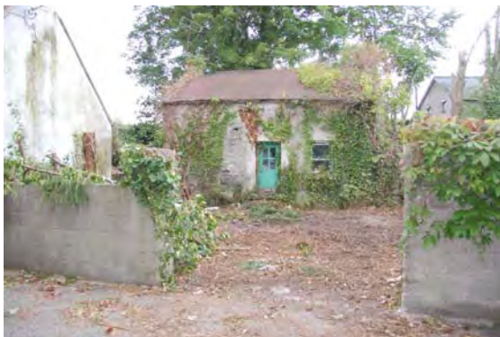
Derelict structures to rear of Main street (Turf Market)
