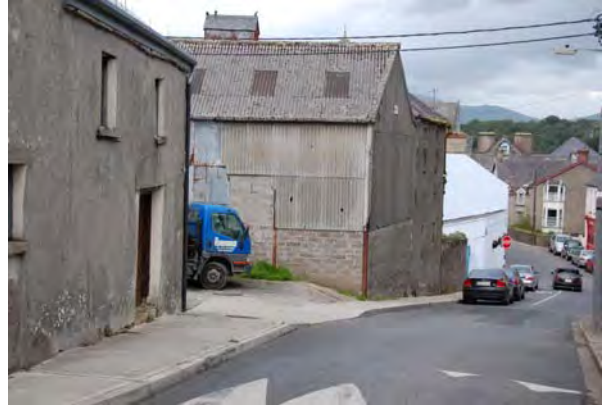
Warehouses on High Street
