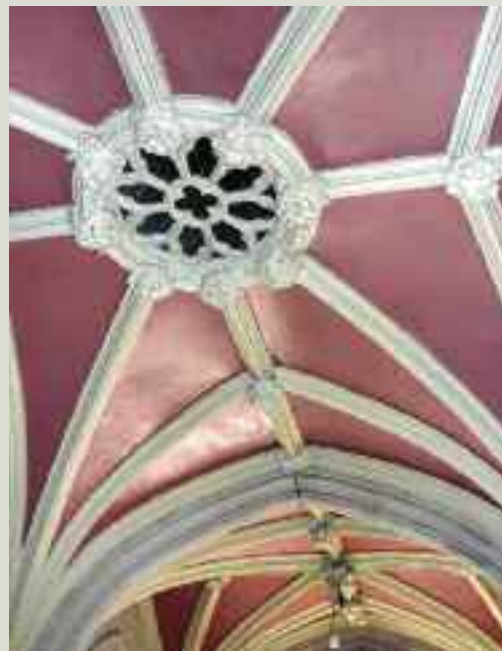
Ceiling grilles should be checked to ensure that the warm, humid air rising into the roof space is ducted through and discharges to the exterior to avoid raising the moisture content of the roof timbers to a level that might make them vulnerable to insect or fungal attack
