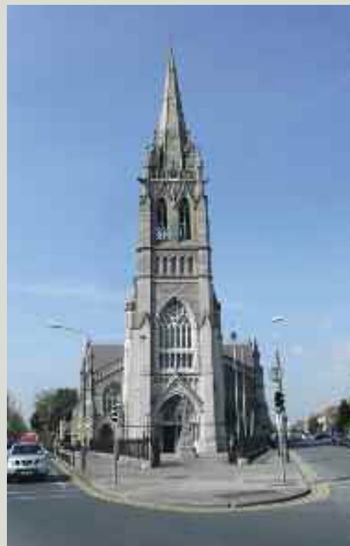
The Roman Catholic church of Saint Peter's, Phibsborough, Dublin has a lofty, cruciform roof and tall steeple, which make roof maintenance a specialised task. Repairs to the roof and guttering were grant-aided in 2009 by the Heritage Council's Significant Places of Public Worship grant scheme
