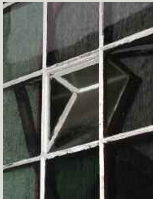
Original ventilators in the glazing should be repaired where necessary and opened after church services. Care should be taken in operating the mechanism to avoid damaging historic glass
