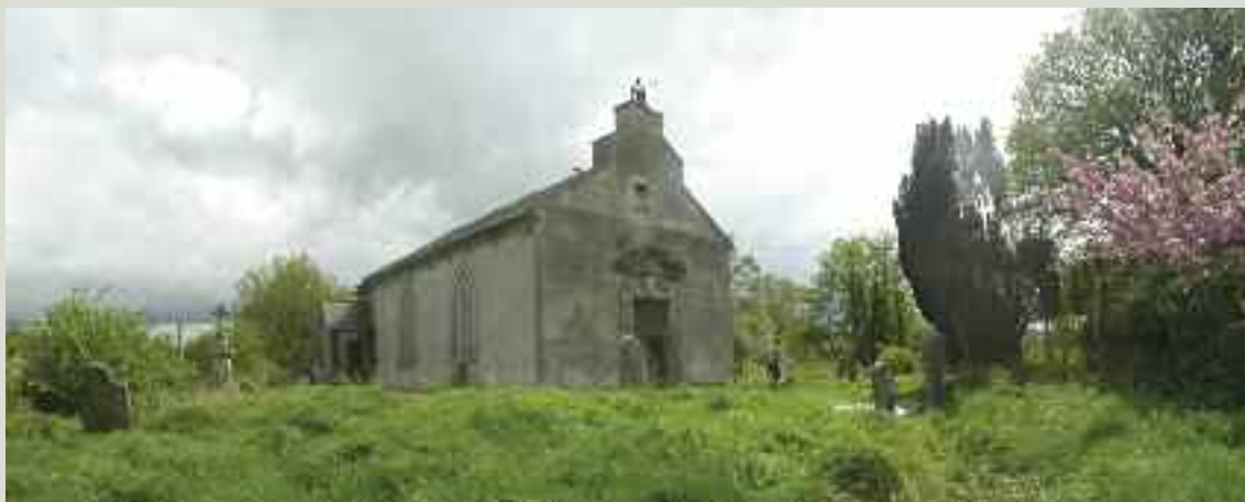
This redundant Church of Ireland church was 'mothballed' to prevent deterioration while decisions are made on its future
